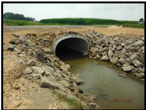
Stentz Road – Elliptical Concrete Culvert
