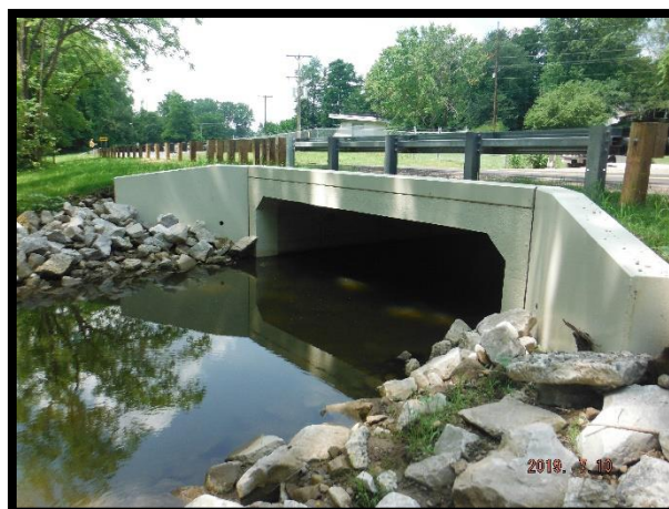
Home Road – Concrete Box Culvert
