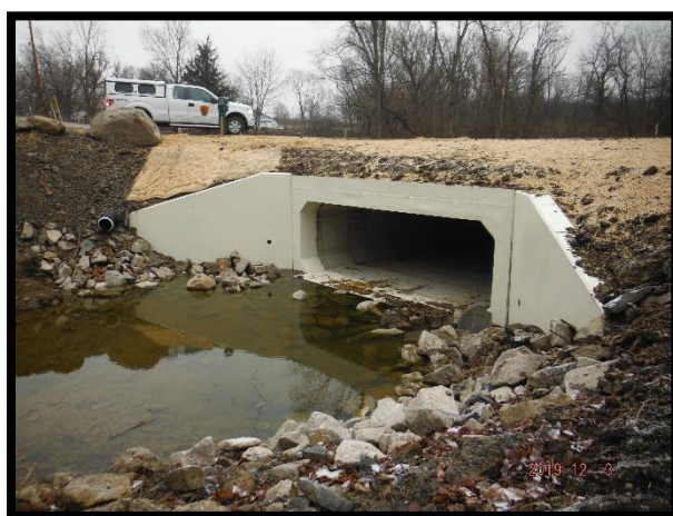
Reynolds Road – Concrete Box Culvert
