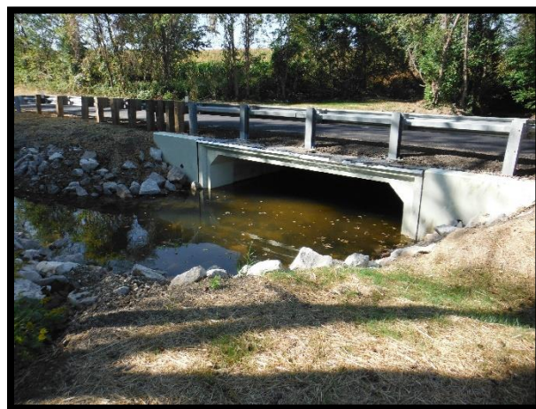
Richland Run Road – Concrete Box Culvert
