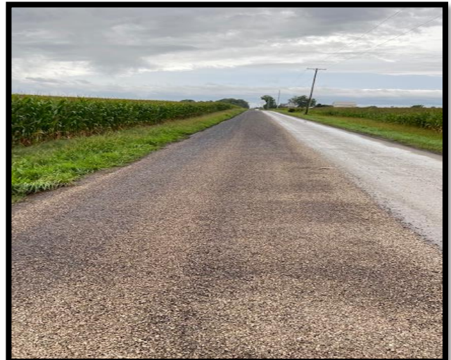
Free Rd – Chip & Seal Resurfacing
