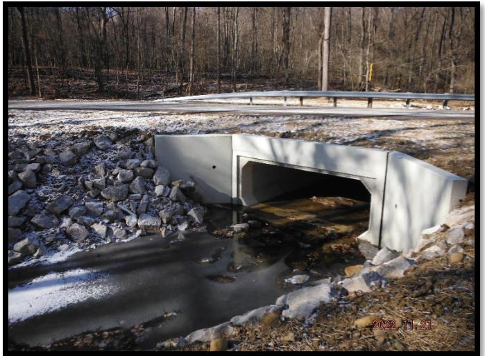
Applegate Rd - Concrete Box Culvert
