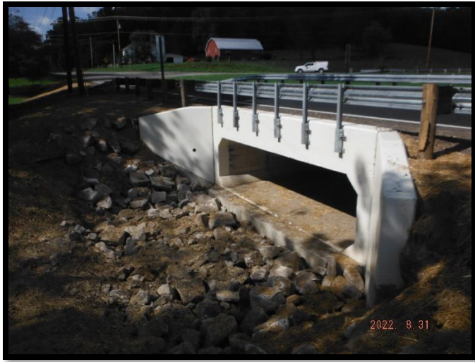
Possum Run Rd - Concrete Box Culvert
