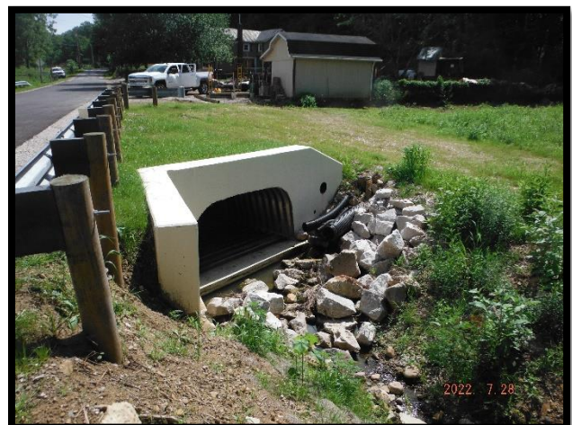
Mill Run Rd – Aluminum Box Culvert
