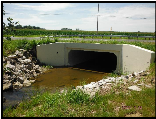
Plymouth-Springmill Rd – Concrete Box Culvert
